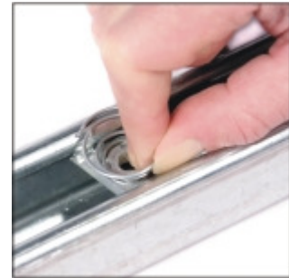
Place in strut and twist
